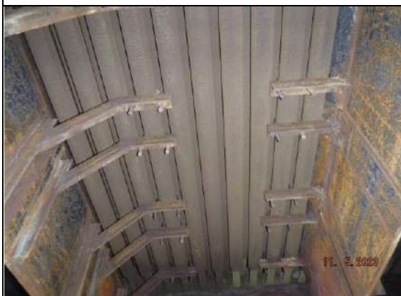
Pic. No. 11 Location : Internal Exhaust Duct
